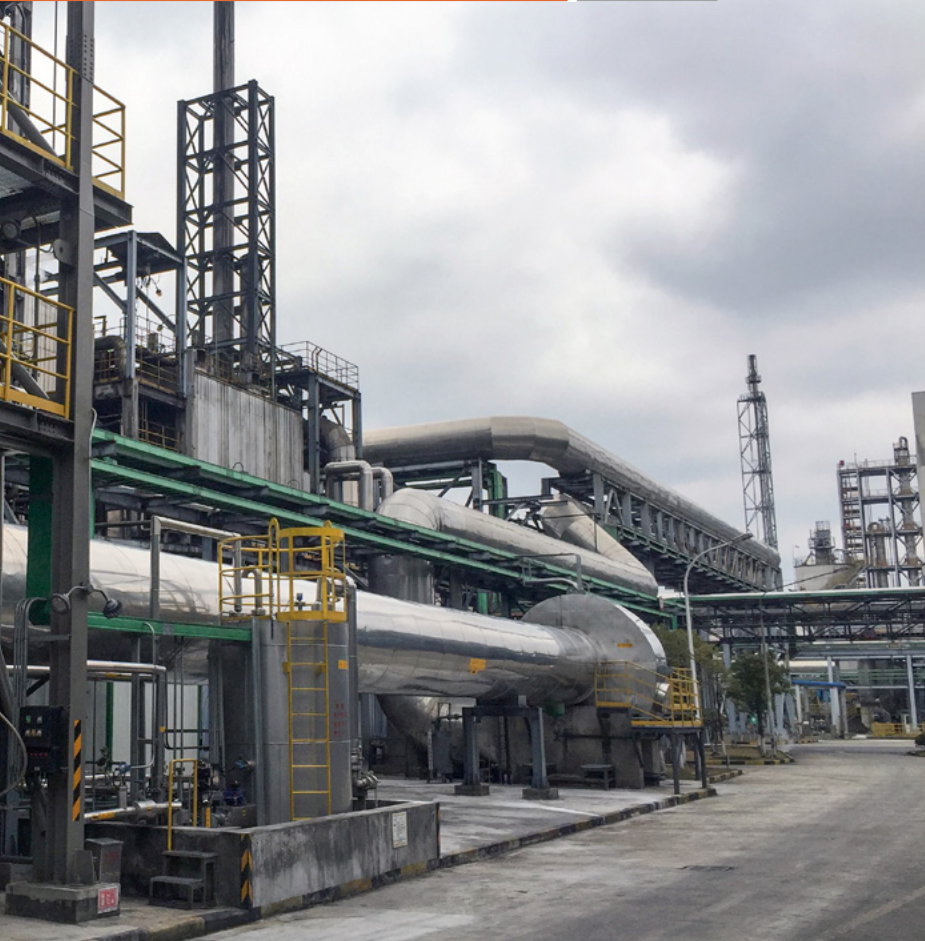
NO x controls in Shanghai, China
